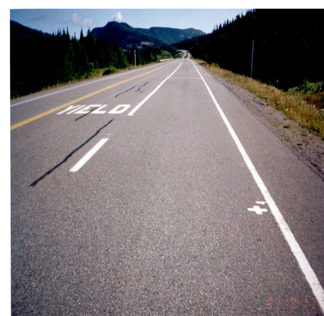
Figure 2: Field Survey of TS 09
